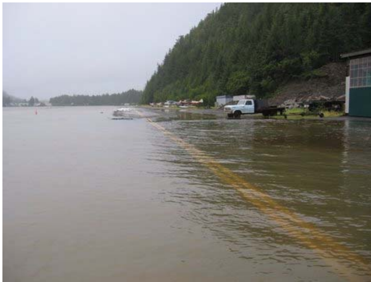
Photo 2: Eyak Lake Airport and other areas along shoreline of Eyak Lake have had some erosion as a result of flooding, 2006.
