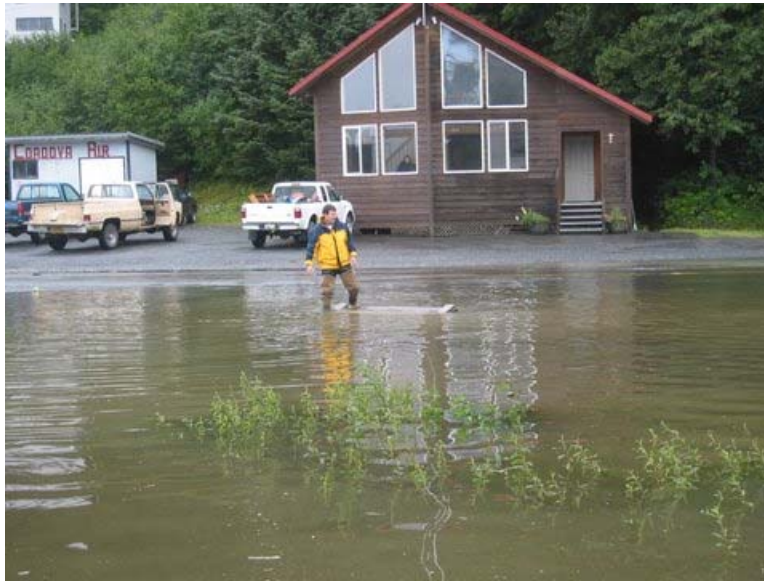
Photo 1: Shoreline erosion near Cordova's Eyak Lake Airport is a concern, December 2002.
